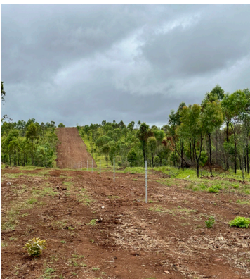
Fencing installed through the GRASS program
